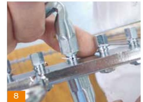
Tighten the wire with the spanner and block the pivot with the nut. Important: the wire needs at least two/three rotations around the pivot before being tense.
