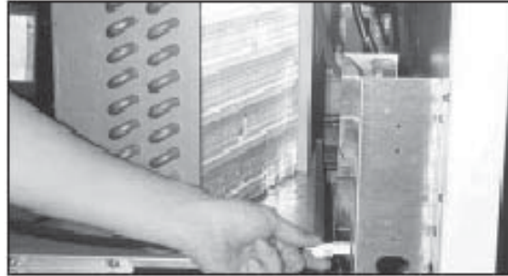
2. Separate the Compressor Harness out of the Switch Box.
